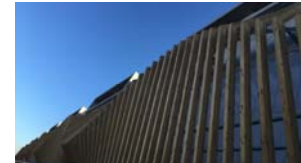
West façade of building
