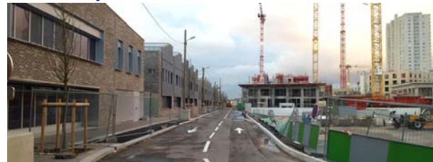
Mixed-use operation, construction site on Chapelle 01/2018
