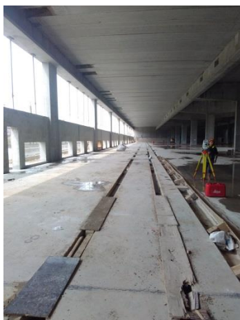
Figure 1. Rail terminal construction at Chapelle.
